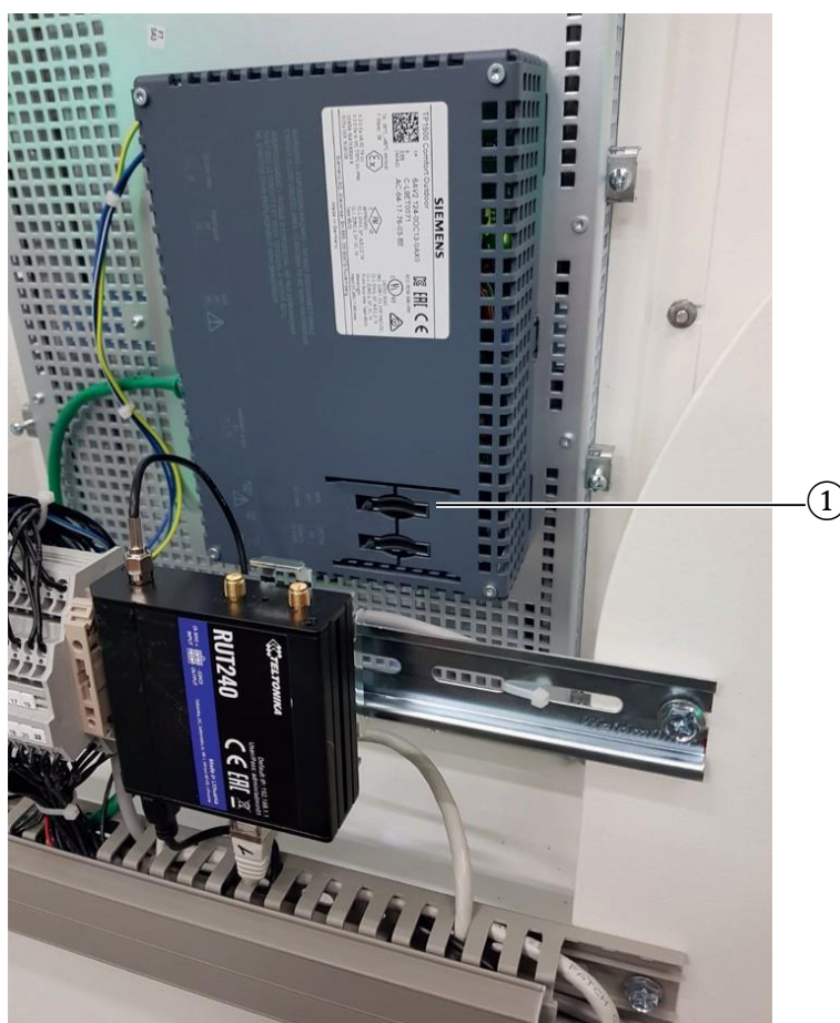
Figure 2-31 ① Position of the slot for the customer SD card
